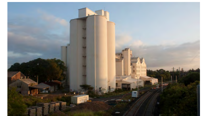
Figure 7.2c: Allied Flour Mill Buildings, Summer Hill
