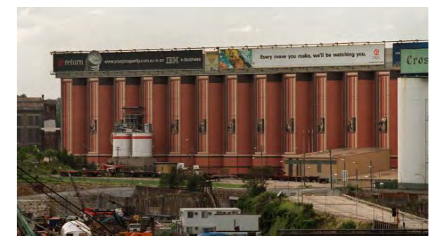
Figure 7.4b: Glebe Island Buildings (source: Website)
