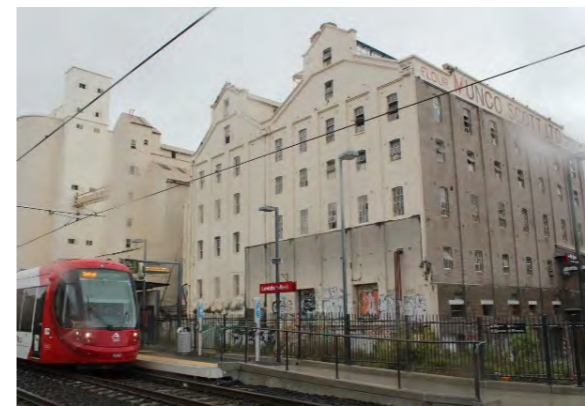
Figure 7.2b: Lewisham Industrial Buildings
