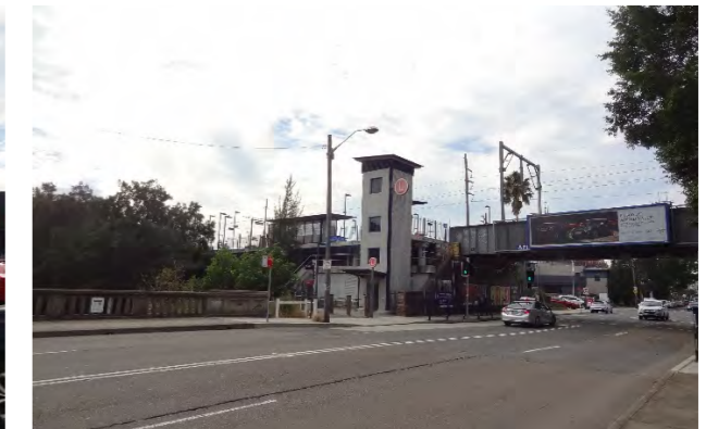
Figure 6.13b: View of Northern Side of Marion Street – from the West to railway bridge and Marion light rail station
