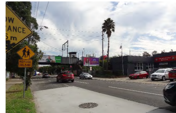
Figure 6.13a: View of Northern Side of Marion Street – to the West to railway bridge
